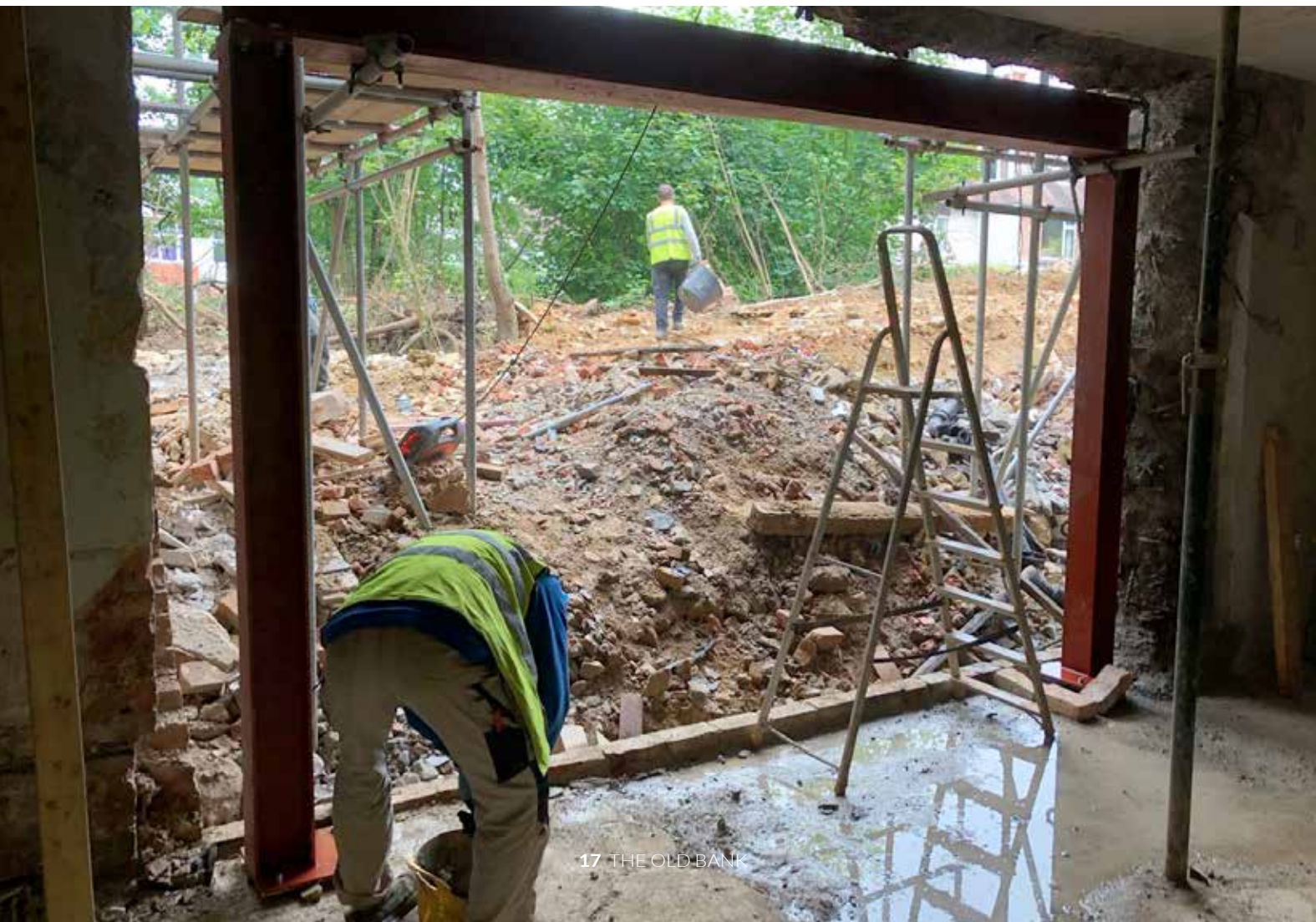
Before New steel frames are being installed.
