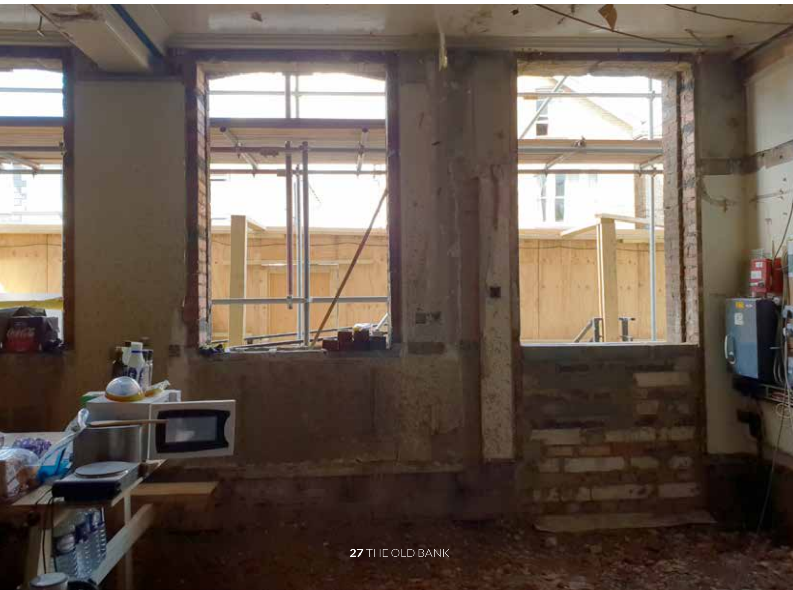
Before The upper floor during restoration works.
