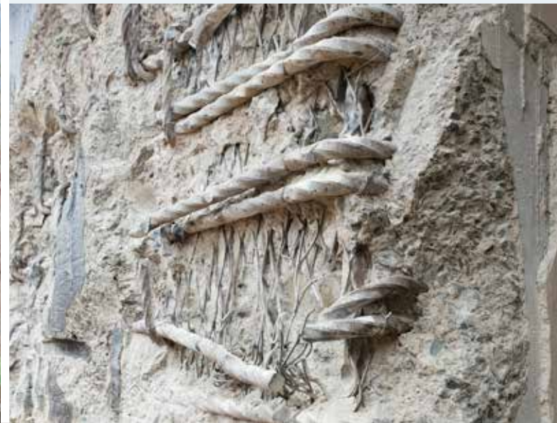
The 1,500mm thick walls of the former vault.
