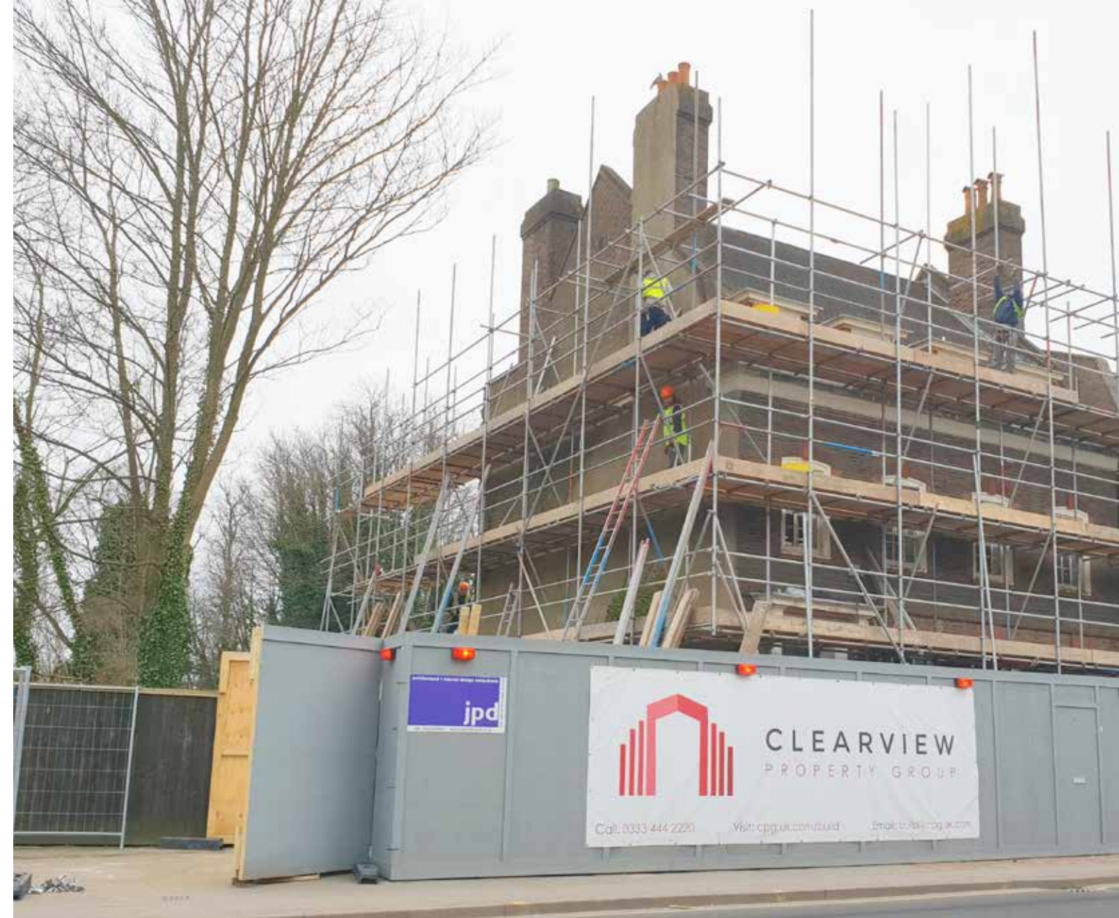
The branded and secured site during construction.
