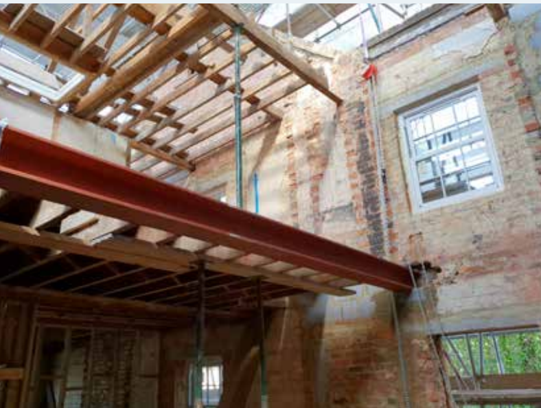
Newly installed steel beams.
